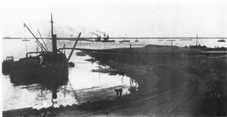
Discharging sand by suction dredges
